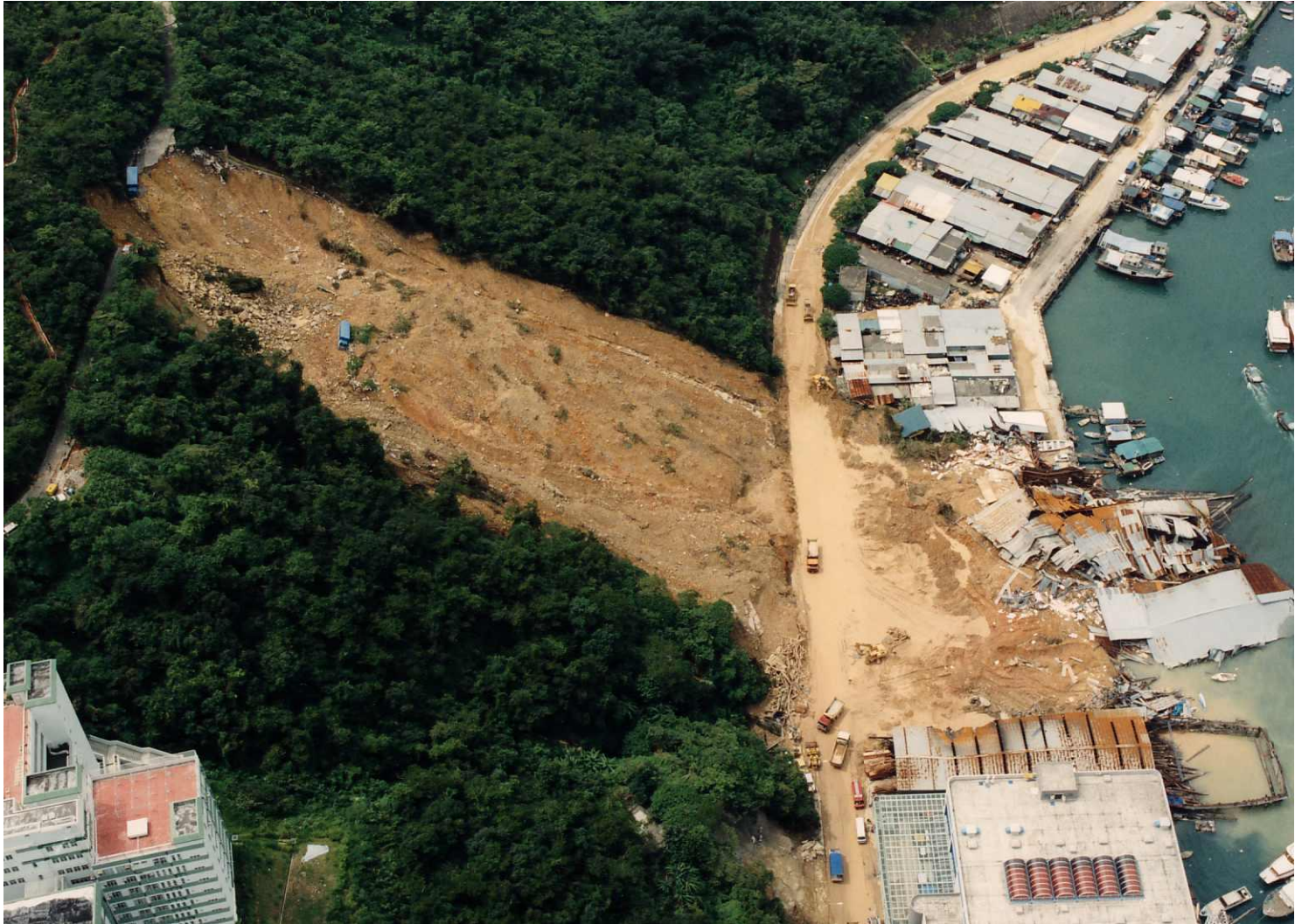
Flowslide in Hong Kong?
